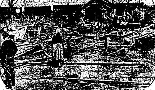
The tremendous task faced by relief agencies in the tornado area of Arkansas is indicated in the picture above, taken at Diaz. Many families lost everything in the storm. Others are, finding their belongings scattered at great distances from their homes.
