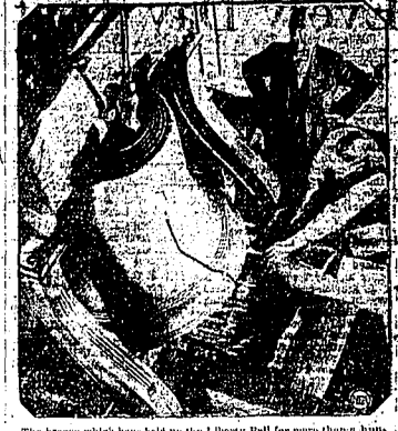
The braces which have held up the Liberty bell for more than a half-century have shown signs of weakness. So new workers are busy in Independence Hall, Philadelphia, and are pictured here installing new supports under the famous bell which "preaches Liberty throughout the land" in 1776.
