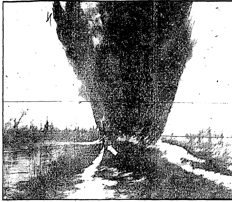
This mighty blast opened a 75-foot gap in the levee near Bird's Point, Mo., above Cairo, Ill., and its accompanying roar was a crashing pean of safety for 14,000 Cairo residents but tremendous signal of disaster for the 35,000 farmers who lived in the 10,000 acres flooded when the gap was opened.
