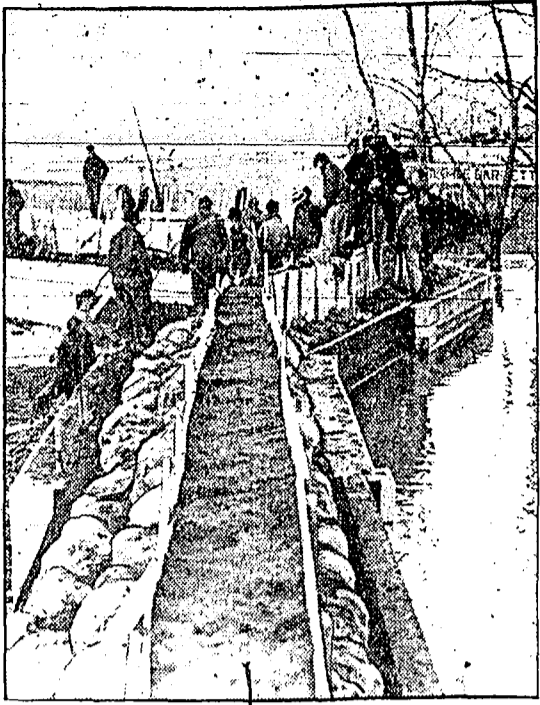
Thousands of workmen labored industriously to add sandbags and build "mud boxes," as shown above, to levee protecting Cairo when flood waters threatened to rise two feet above the permanent floodwall. "Mud boxes" are built by filling a framework of timber with cinders and earth, sometimes for miles.
