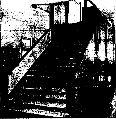
Here is the most serious fire menace in the Twin Falls school system as it now exists—the open central stairway at the 20-year-old Bickel building. Authorities declare the open stairway would act as a dangerous fire in case of fire, and would permit flames to sweep upward through the building in a few moments, with the danger of trapping hundreds of youngsters. The new Bickel Building under the proposed school bond issue would replace the present structure and remove the fire hazard.
