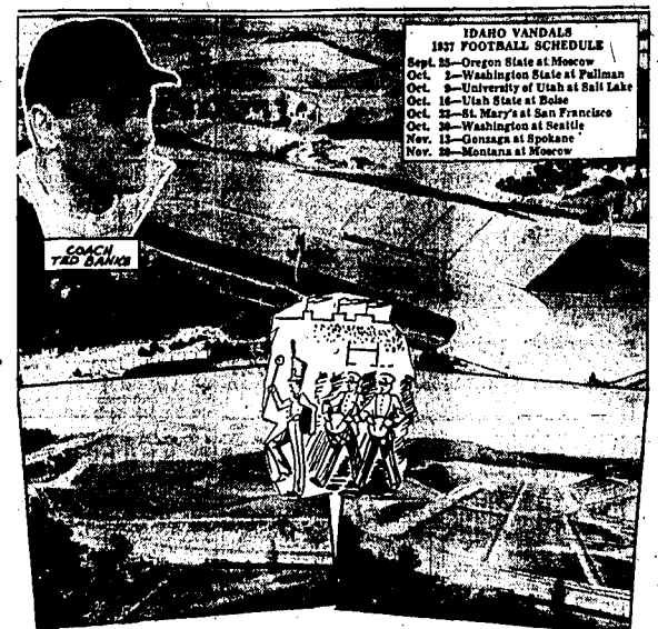
With the completion of the new Neale stadium at the University of Idaho, Coach Ted Banks, athletic director, started his Vandals on grid practice with an optimistic eye. Pictured above are the stages of construction of the new stadium. Lower left photo shows the plot of ground as it stood a year ago before excavation started. Lower right shows the structure after the excavation had been completed and the frame work for the seats was placed. At the top is the artist's conception of the completed structure.
