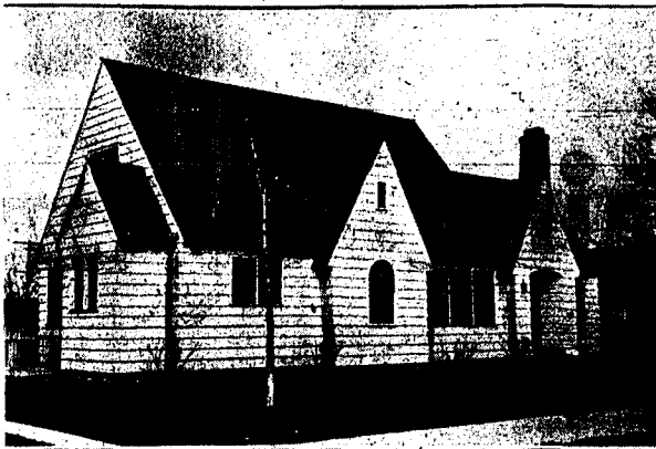
The residence of Mr. and Mrs. Guy H. Shearer (pictured above), at 1121 Tenth avenue east, is one of the homes which has been completed recently in Twin Falls. Insulated throughout, the home is cool in summer and warm in winter. Shrubs and new trees add to the beauty of the structure during the late spring and summer months. (Evening Times Staff Photo.)
