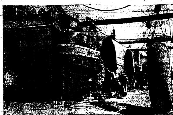
The snow cruiser built in Chicago for the U. S. Antarctic expedition, dwarfs the men beside it. One of its 16-foot, half-ton wheels is shown.
