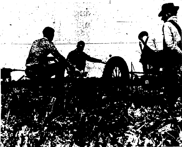
As an interested farmer (right), one of more than a score who witnessed the demonstration, looks on, the new sugar beet topper is "put through its paces" for its first Idaho test. The new machine, still in the experimental stage, is being perfected by the University of California. In the above picture, taken yesterday during the field demonstration, John Powers (left) and Roy Barker (center), both of the University, are shown as the test started. On a small tractor which pulled the new machine is Herman Huff of the Annapolis Sugar company. The machine is designed to top the beets while they are still in the ground. The test took place in a field near the local sugar factory, where a second new device was also tried out. That machine is handled by a commercial firm. (Times Photo and Engraving)
