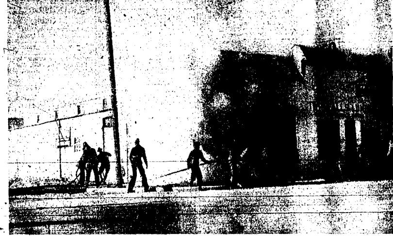
With fire hoses stretched from various hydrants to the blaze, local firemen and volunteers this morning had their hands full as a brisk, cold wind aided the flames which spread through the Twin Falls Lumber company building here. The fire started at 10:15 a. m. and it was 28 minutes before the "under control" sign was given. In the picture above, taken as the firemen started their work, regulars and volunteers can be seen shifting hoses to strategic positions. Smoke is drifting to the right from the structure, as the fire rages to the left and of the picture toward the roof. Volunteers had not yet started removal of store equipment before this picture was snapped. After this photo was taken, the fire was placed against the structure and firemen succeeded in the roof.
