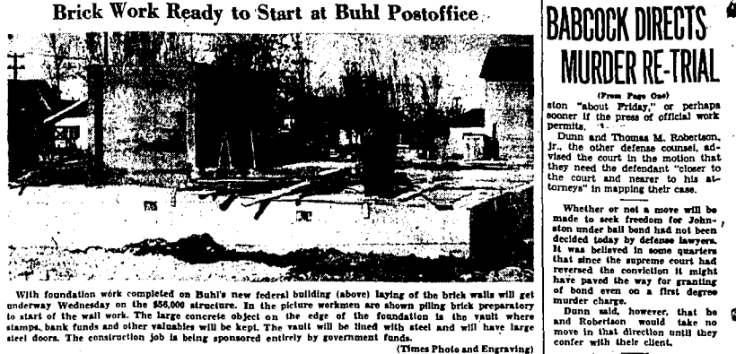
Brick Work Ready to Start at Buhl Postoffice
