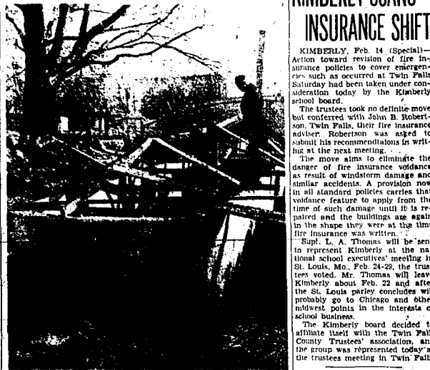
In connection with construction of the swimming pool at the Buhl city park, other construction is being carried on at the present time. Above, workers are shown preparing the ground in preparation for the concrete work which will get underway as soon as weather permits. A chlorinating plant will be placed under the sidewalk near the concrete structure visible near the center of the picture. The pool itself will be 124 by 68 feet.
