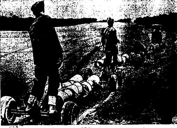
Even with cushiony balloon tires on the "carr," British aircraftmen acting as "conductors" on this deadly train are glad the field they are crossing is fairly flat. The tractor-drawn train consists of loaded bomb-carriers.
