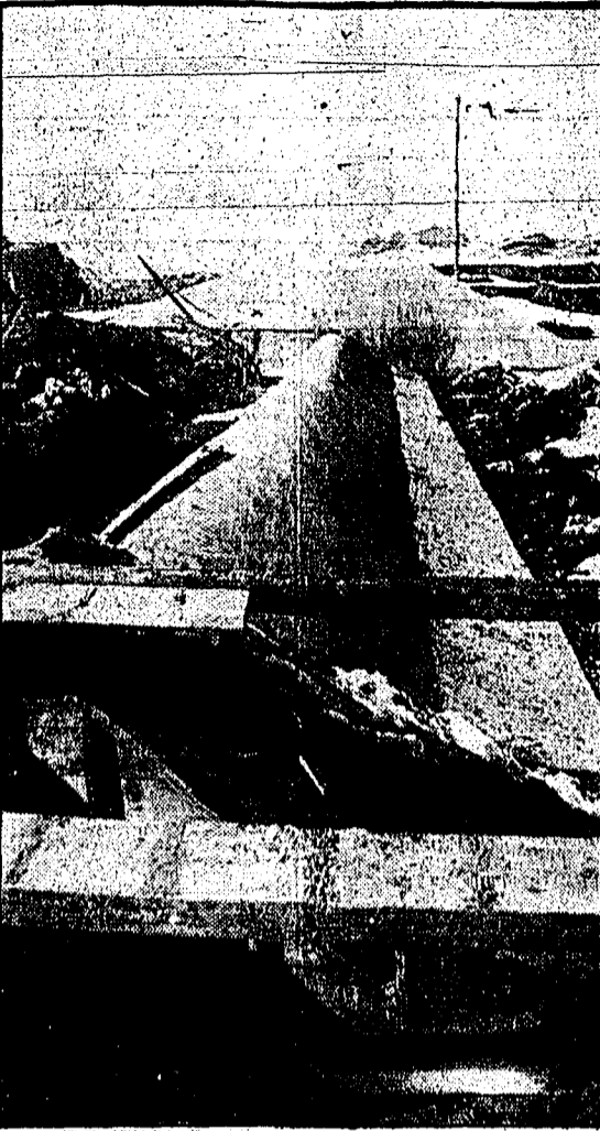
Shown above is a section of the concrete spillway at the Little Wood river dam near Carey. Construction work on the dam, which will result in its completion in a period of some five months, is expected to resume by June. When WPA work on the dam stopped, farmers of the district threatened "armed protest" unless provision were made to complete it. Water which it would impound is vital to the welfare of hundreds of Idahoans cultivating from 6,000 to 8,000 acres. (Times Engraving)
