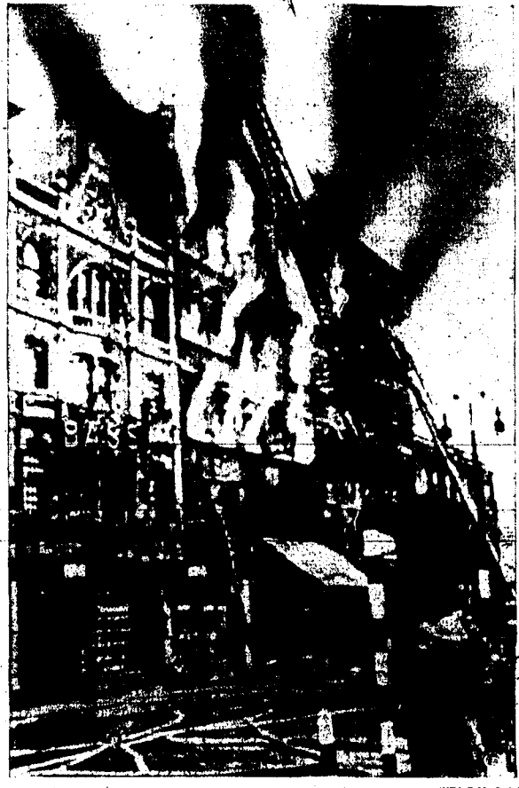
Raging flames from incendiary bombs gut a building in central London following the merciless "all-out" raids of Sept. 25. This scene, captured from London, was being duplicated in many sections of the great city—heart of the British Isles.
