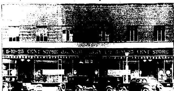
Outside view of the new J. J. Newberry store which opens in Twin Falls Thursday shows the impressive nature of the building reconstruction which preceded the grand opening. The front adds another modernistic note to a Twin Falls business district which is rapidly becoming one of the most "streamlined" in the intermountain area. (Times Photo and Engraving)
