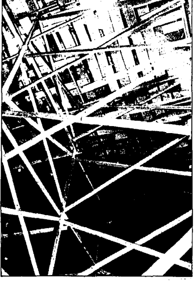
This may make you dizzy but it's a matter of news because it's termed the largest interior scaffolding ever erected in Magic Valley, and one of the largest in Idaho.
