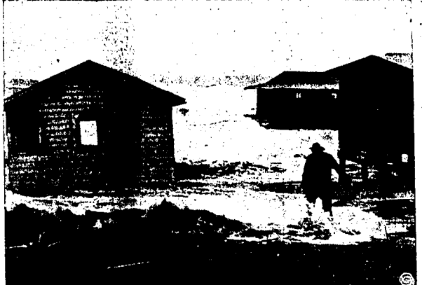
Large breakers curl around undermined and toppled beach cottages at Suisun beach, near San Francisco, during high tides and heavy winds that caused extensive damage.
