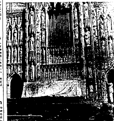
With much of the delicate Gothic sculpture already in place, work is being rushed to have the magnificent high altar finished in time for Easter services.
