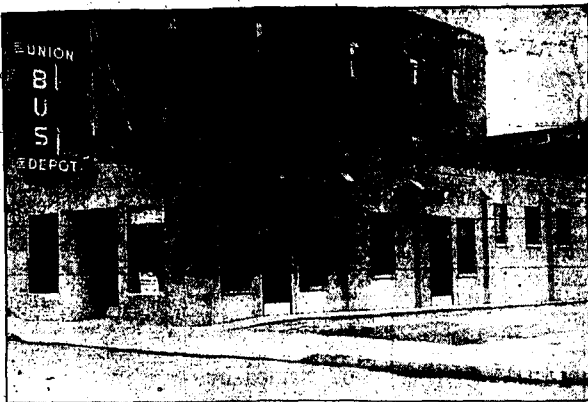
Above is an exterior view of the new union bus depot which will be dedicated here Saturday during a program set to start at 12:15 p. m. Stage company and city officials will participate. Contractor on the new station was Ernest White, Twin Falls, and cost was placed at $20,000. It is located at the corner of Second avenue and Second street east. (Times Photo and Engraving)
