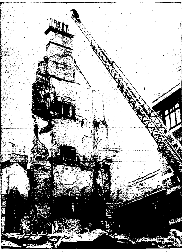
Spectacular picture illustrates one of tough jobs left for Londoners after the bombers have gone. A demolition worker goes way up there on a giant crane to fix steel cables to the wall of what was once a building before remains are pulled down.
