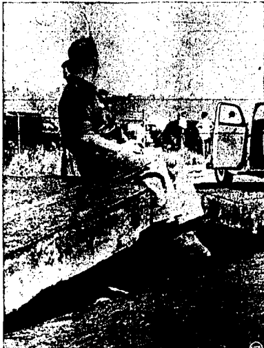
Towns where eggs are "fried on the sidewalk" had nothing on Seattle, Wash. the other day when a scorching heat wave caused two paving blocks to swell, rise in the air and block two lanes of traffic. A workman, above, perches on the inflated "v."
