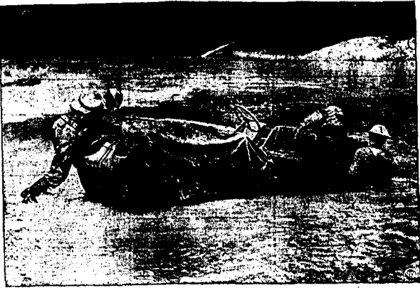
In line of bridgework, the mahouts of a motorized division float vehicles wrapped in canvas across a stream near Fort Benning, Ga. This 500-pound car was pushed onto canvas spread on the water, tucked in snugly for a dry jump to the other side.
