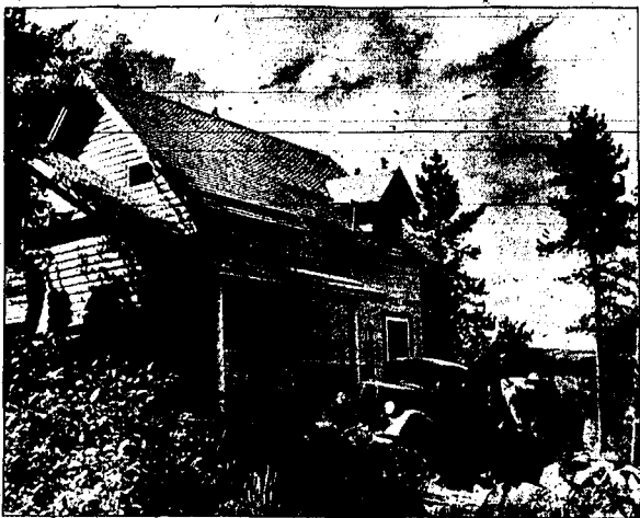
It was a holiday for most people yesterday, but not for 10 members of the Presbyterian church men's club and an equal number of Boy Scouts who worked on the Scout cabin (above) now being constructed in Bates gulch, near the Magic mountain ski area, up Rock creek. The two-story structure will be completed in about 30 days and is for use of members of troop 66, sponsored by the men's club. The cabin is being completed mostly by volunteer labor under the direction of D. R. Young, chairman of the troop committee. The truck shown is being used to haul rock for the large fireplace which will be one feature of the cabin.
