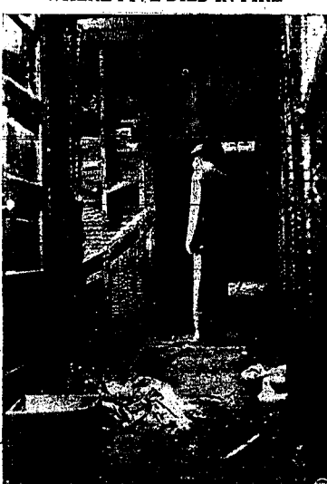
It was on this stairway landing that five of the seven victims of a San Francisco rooming house fire met death. The stairway acted as a draft, and the inmates were cut off from escape. Twenty others were injured.
