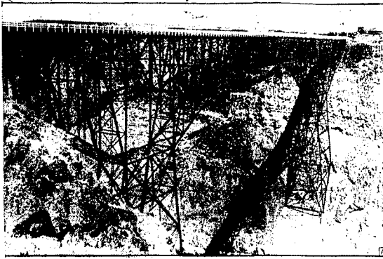
TWIN FALLS-JEROME intercounty bridge, spanning Snake river canyon, is to be operated under toll under provisions of a one-year lease and option which representatives of the state and bridge company signed at Boise late yesterday. Tolls collected since completion of the bridge in September, 1937, have approximated $70,000 a year.
