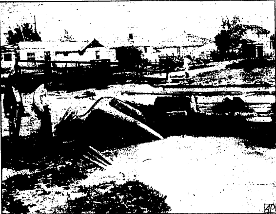
SUDDEN floodwaters following cloudburst rains caused thousands of dollars of property damage along the Milk river in north central Montana, besides taking nine lives and leaving one person missing.
