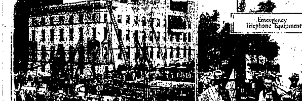
Cleveland Clinic Building During Rescue Work
