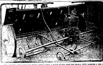
This movable armorprotected shield, behind which a squad of men could find sheller while pumping a rain of shells into the genmy, is one of many being used by the Germans. It is the invention of the Russians, who made use of it when the Germans were laying alego to the flussian fortreas at Grodow. The apparatus is equipped with six wheels. Two horses are harmessed to it is order to bring it into position.
