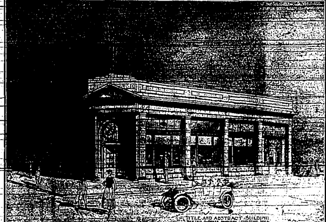
Modern office building of white terra cotta and plate glass front to be built on corner of Shoshone street and Second avenue east. The plans were prepared by Architect Morse, and construction is to begin immediately.
