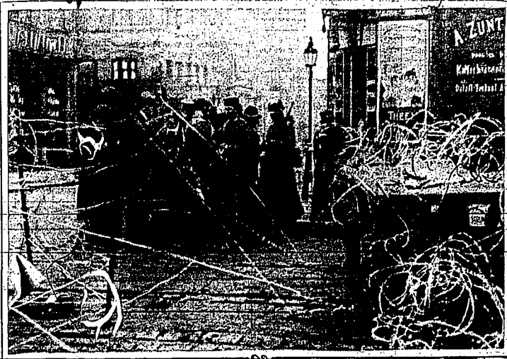
Barbed wire entanglements have been set up in Berlin streets to keep the Bolsheviks back and if another uprising of them occurs the fighting will resemble that on French and Belgian battlefields. This picture was one taken in one of Berlin's principal streets, and is the first to be received in this country.
