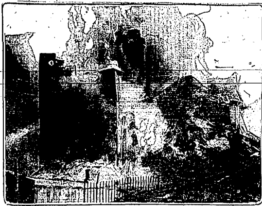
Away went a billion loaves of bread—or perhaps a little less—when this Pittsburg grain elevator went up in smoke, and wheat going up! A large quantity of grain had been stored in its bins. Two firemen were hurt when the walls at the right fell in.
