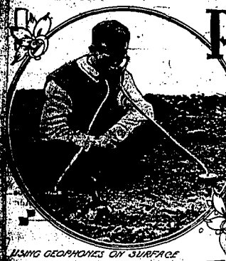
USING GEOPHONES ON SURFACE
