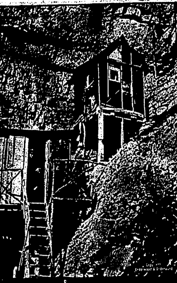
High on the sides of the mountains where they are battling the Austrians and Germans above the clouds in the land of mountains, the Italian troops have built these unusual structures stuck out of sight and reach of the German gunners. Ladders of wood lead up the cliffs from the shelters on the very top. The huts themselves are built on stilts wherever the ledges of rock permit sufficient space for the foundations. The ones shown here are used by a lookout post.
