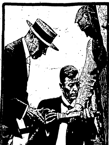
President Wilson is here seen driving the first rivet in the keel of a 10,000-ton cargo carrier, this being the first keel to be laid in the steel shipyards at Alexandria, Va.
