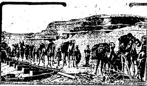
transport attached to the British army crossing a puntion bridge, built by British engineers acrossing a function. The transport is in the rear of the British army which has routed the Torks out of Palestin
