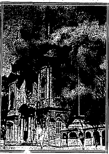
Estimating a loss of approximately $1,500,000, the historic Church of Saint Anne De Beaugrand in Quebec, Province of Quebec, Canada, was almost destroyed by fire. Some of the most sacred relics in the Western hemisphere were housed in the famous edifice...
