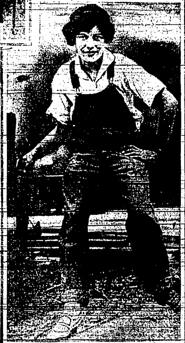
CARPENTERING PAYS —Mrs. Florence Worden is the first full-fledged carpenter in a Miami suburb. With her hammer and saw she supports herself and sends her son through a Southern military academy. (International News)
