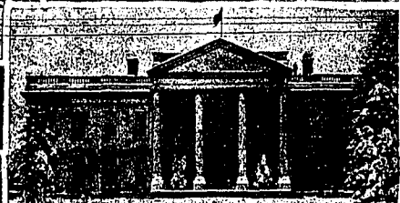
WHITE HOUSE ROOF WEAK —Fear that the White House roof might collapse was expressed by Major U. S. Grant, 3rd, supervisor of public buildings. Heavy snows this winter have strained the ancient structure considerably. (International Newsreel)
