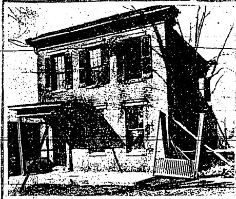
MIDDLE-WEST TORNADO —One of the buildings wrecked by the wind that tore through Hannibal, Mo., after leaving a wake of disaster in Oklahoma, Missouri and Texas. The occupants escaped.
