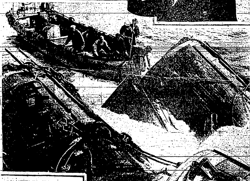
S-51 LIFTED TO SURFACE —The nose of the S-51 appeared above the surface of waters off New London, Conn., for the first time since it was sunk in a crash on September 28, 1925. Salvagers encountered difficulty, and the submarine and supporting balloons were lowered to await another try. (International News)
