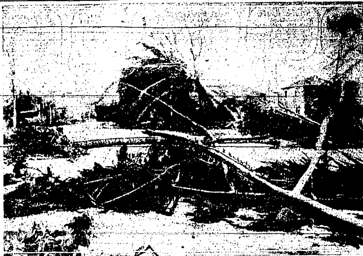
ALONG BEAUTIFUL MIAMI BEACH where green-fronted trees lined the shore and semi-tropical vegetation lured the tourist to their grateful shade here is now a barren desolation. The trees are lying flat and dead in three feet of water that backed up for four blocks. Behind them are ruined houses. Picture telephotographed by International News Service.
