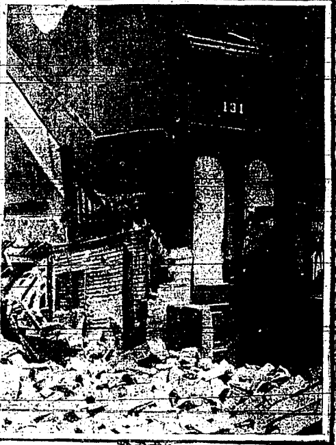
A DOOR...BUT THAT'S ALL —A nearby excavation caused a four-story building to collapse in New York, leaving only the door standing. Tenants were warned in time to flee. (International Newsreel)
