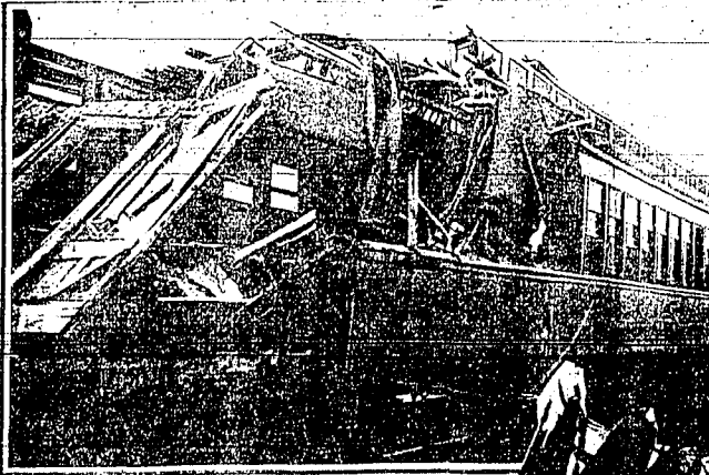
VACATION JOYS END IN DEATH —A train, burdened with returning vacationists, collapsed with a freight train at Long Island, N. Y. Five persons were killed and almost sixty injured. (International Newsphoto)
