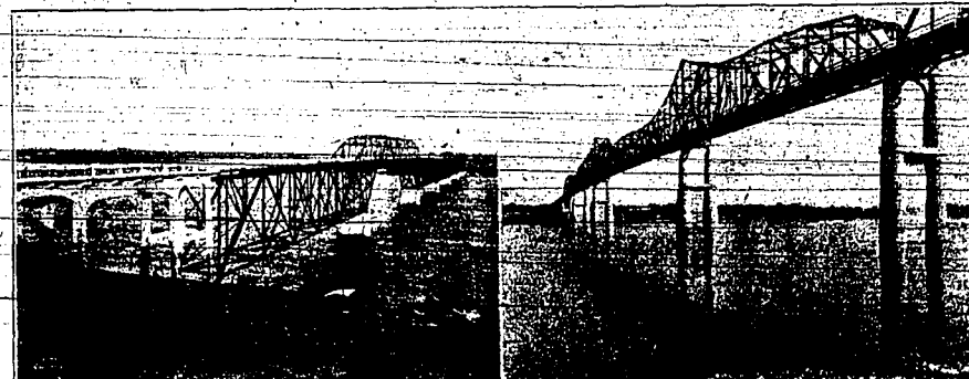
UPPER LEFT—The Pasco-Burhank Bridge over the Snake River, length, 1,500 feet; height, 75 feet above low water; channel span, 300 feet. Opened for traffic in 1921. UPPER RIGHT—Pasco-Kennewick Bridge over the Columbia River; length, 3,200 feet; longest span, 420 feet; height above the low water, 75 feet. Opened for traffic in 1922. LOWER LEFT—Bridge of the Gods over the Columbia at Cascade Lock, Oregon. 700 foot span; 150 feet above the river; total length, 1,400 feet. Opened October 1926. LOWER RIGHT—Cowlitz River Bridge, Olegus, Washington. Length of structure 500 feet. Opened for traffic in 1925. All designed by the Union Bridge Company, Portland, Oregon.
