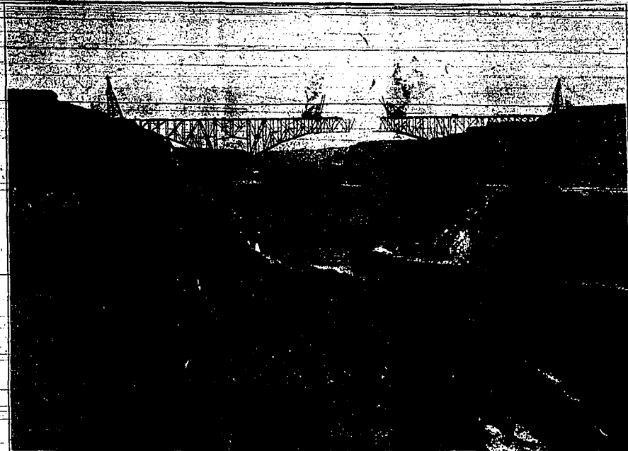
THE PICTURE SHOWS the method of construction employed in the building of the cantilever type of bridge. The final joining up of the two ends took place just a few days in advance of the opening, September 15.
