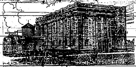
Idaho Power Company's Substation at Boise
