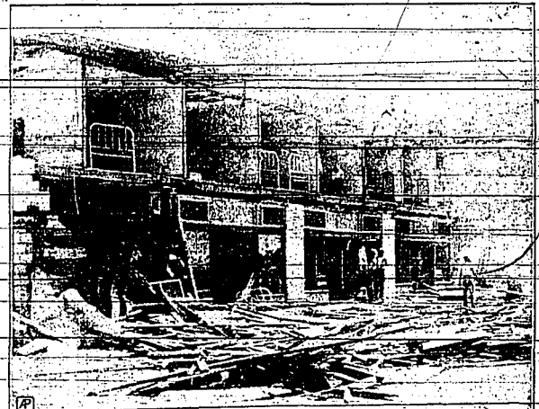
ALTHOUGH THE FURNITURE in these hotel rooms was undisturbed the entire east wall of this West Palm Beach hostelry was carried away when the tropical hurricane swept the town.
