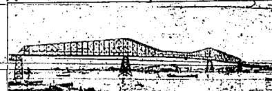
DRAWING OF $5,800,000 structure which will connect Longview, Washington, and Rainier, Oregon. It will have a clearance of 195 feet, a center span of 1200 feet and, with approaches, will be a mile and a half long.
