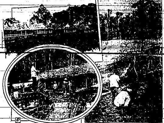
Modern bungalows (upper left) have been erected for overseers on the Ford rubber plantation in Brazil. At the right, natives are clearing the jungle. The density of the growth is indicated in the distance. At lower left is a sawmill on the plantation.
