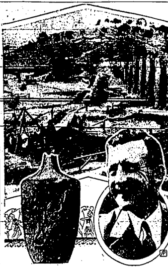
Above, the work of paralleling a section of the ancient Hadrian aqueduct with steel pipe to increase the water supply of Athens. The task is directed by R. W. Gausman (lower right), American engineer. At lower left is a Grecian urn dating from 300 B. C., found by workers under Gausman.
