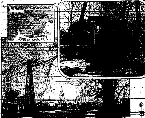
American capital is introducing deep drilling and modern machinery into German oil fields where, as shown, clumsy beam pumps topped by old-style tripods, now raise small amounts of petroleum.
